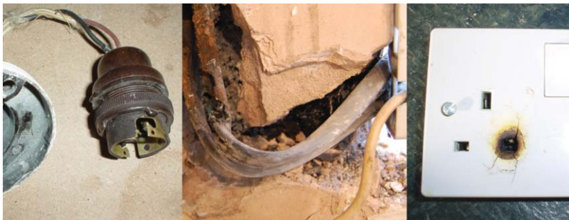
▲ Typical examples of potentially dangerous electrical installations
